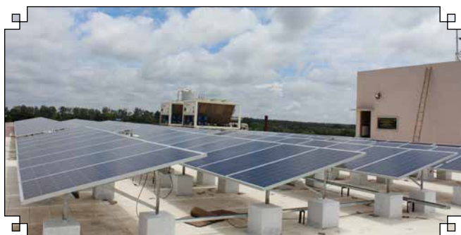
Solar panel (50 kw) has been installed on the roof top of the Laboratory Building
